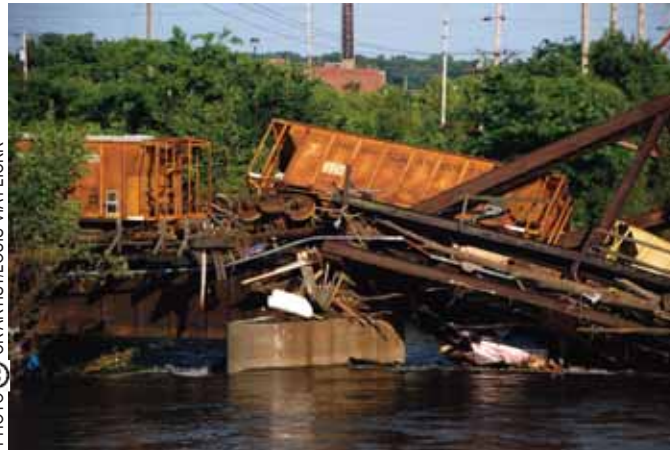
Collapse of the Cedar Rapids and Iowa City (CRANDIC) railroad bridge during June 2008 flooding on the Cedar River in Cedar Rapids, Iowa.
