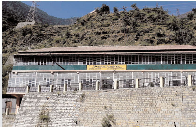
The Larji Project office complex rises above the river and across the highway from where the students drowned. Photographer: Tom Lasseter/Bloomberg
